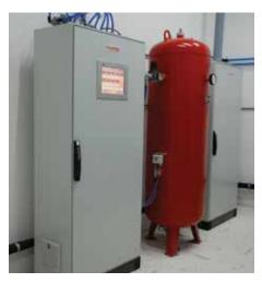
Two standing cabinets for generator and distribution system with inbuilt control unit and separate hypoxic air buffer vessel
