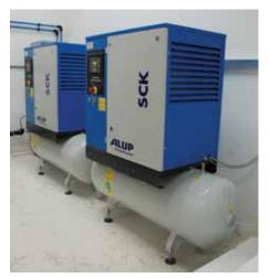
Two compressors on buffer vessels
